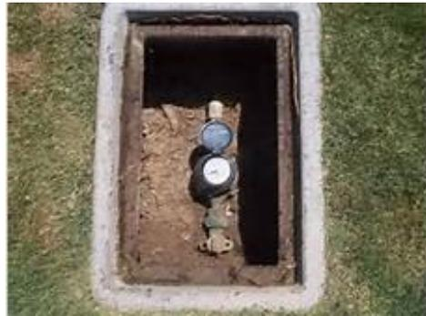
The meter is usually in a plastic or cement rectangular box flush to the ground with a small hole in the top of the box, normally located close to the street and/ or sidewalk or alley close to your property line. The number of the meter should match the meter number on your water bill.
