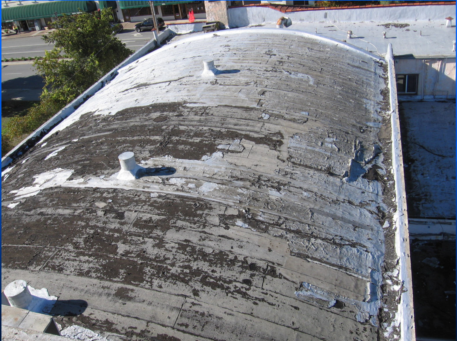
Auditorium "Barrel" Roof looking West
