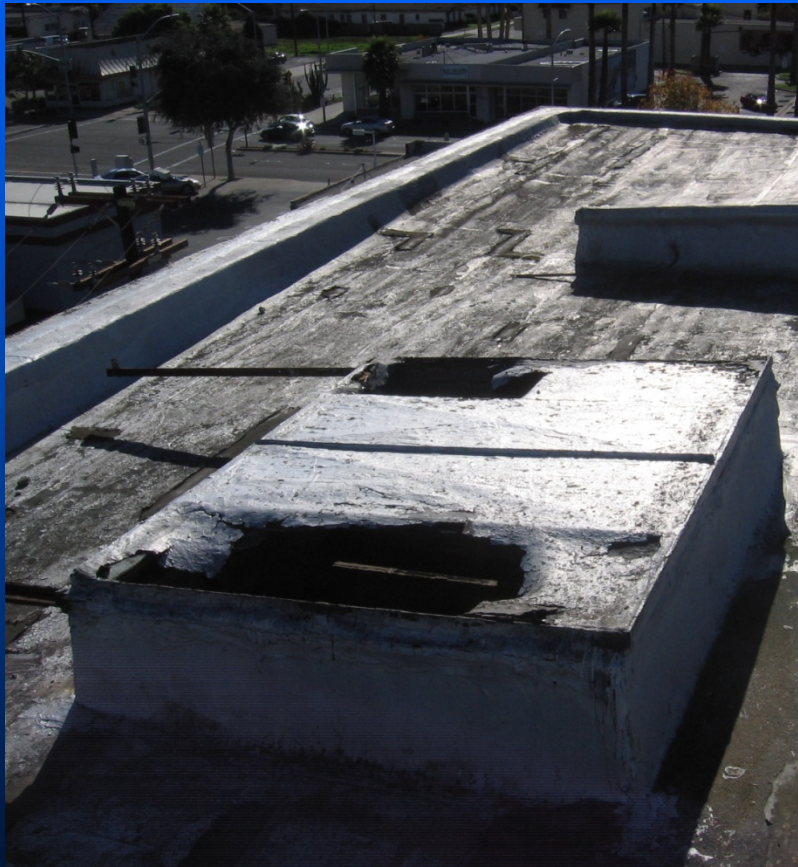
Fly-Tower Roof over Stage
