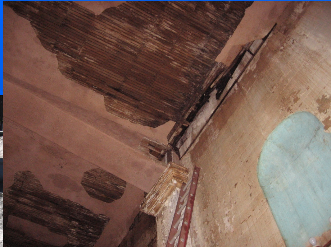
Auditorium Ceiling at South Wall
