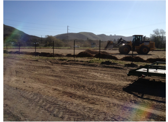
SETTING THE FENCE POSTS AND CREATING A BERM OF WOODCHIPS FOR SAFETY
