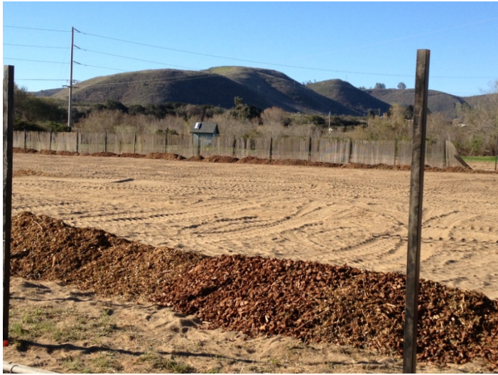
SETTING THE FENCE POSTS AND CREATING A BERM OF WOODCHIPS FOR SAFETY
