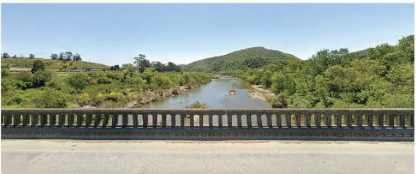
EXISTING BRIDGE BARRIER
