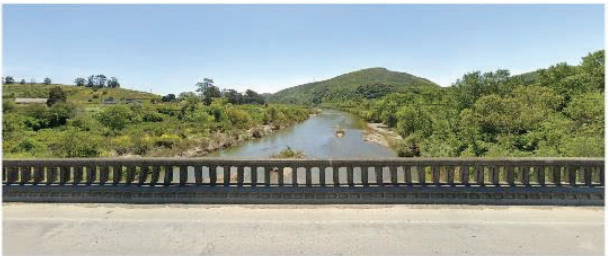
EXISTING BRIDGE BARRIER
