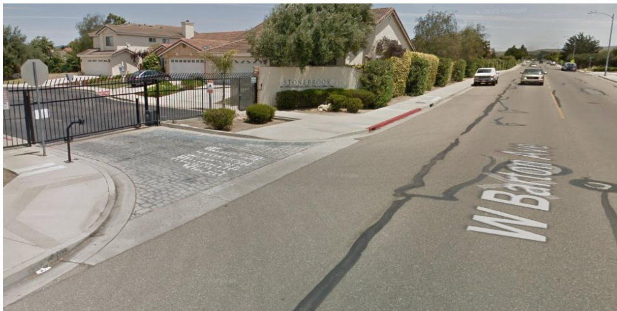
Figure 5 - Stonebrook Ped & Veh Gate - Barton Ave
