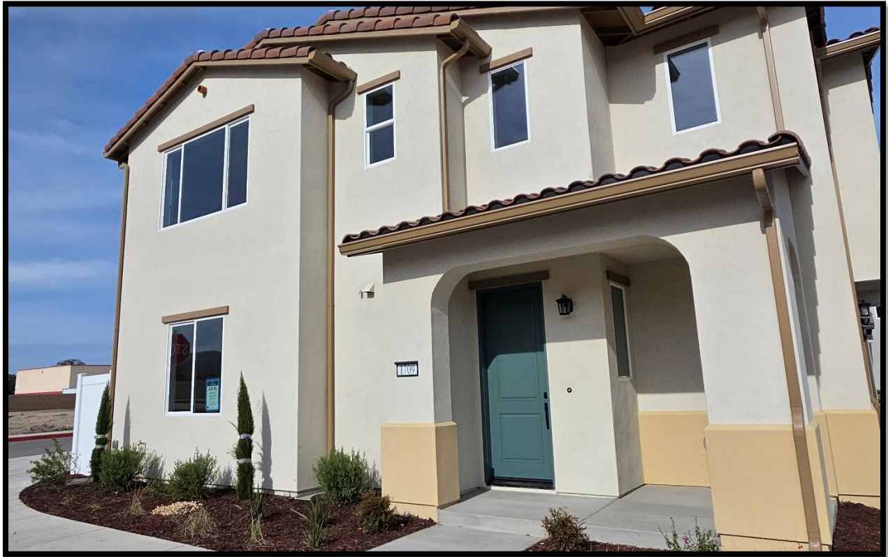
Source: New homes at the River Terrace Development taken by City Staff, December 2025
